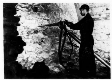
WUP-20 PNEUMATIC HAMMER DRILL with air-water flushing mounted on a PWU-51 airleg pictured in a Soviet Orbit demonstration mine. Weight of drill is reported as 49.6 pounds and the airleg 47.4 pounds.
